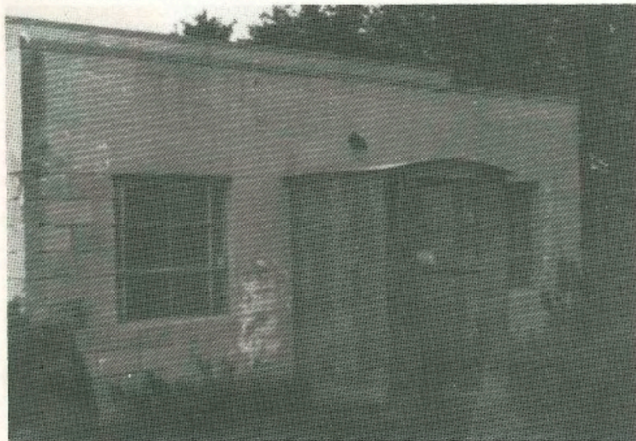
The Water District office before it underwent remodeling this year.
