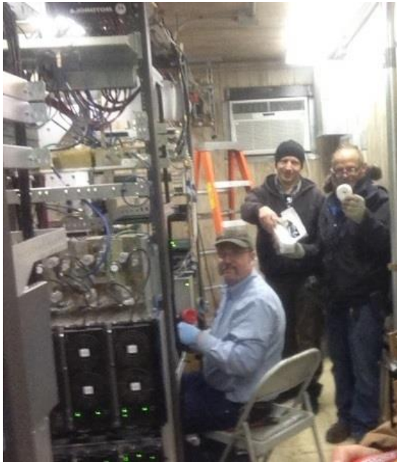
From left to right: Joel, Marty and Jim doing the technical installation.
